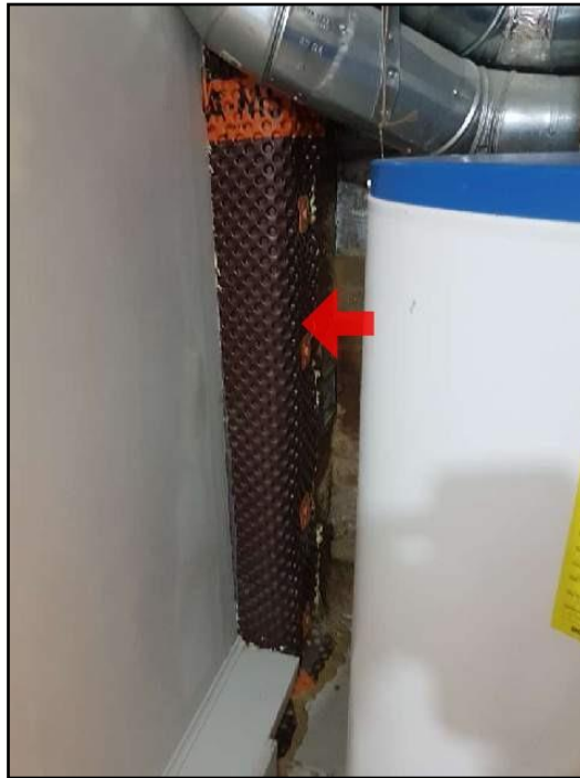
10. Interior drainage membrane.
