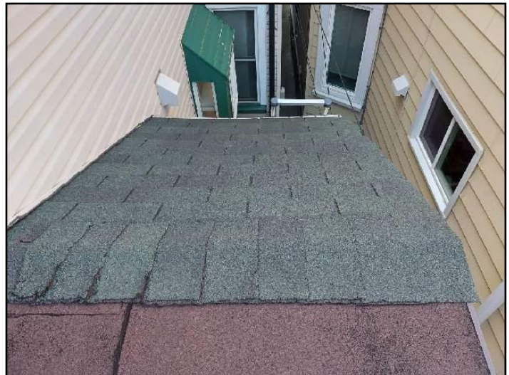
5. Replace ridge cap
