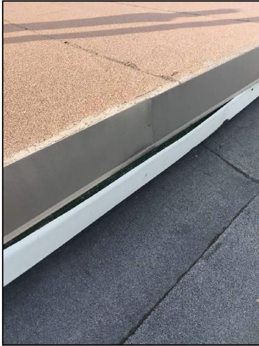
6. Secure loose flashing
