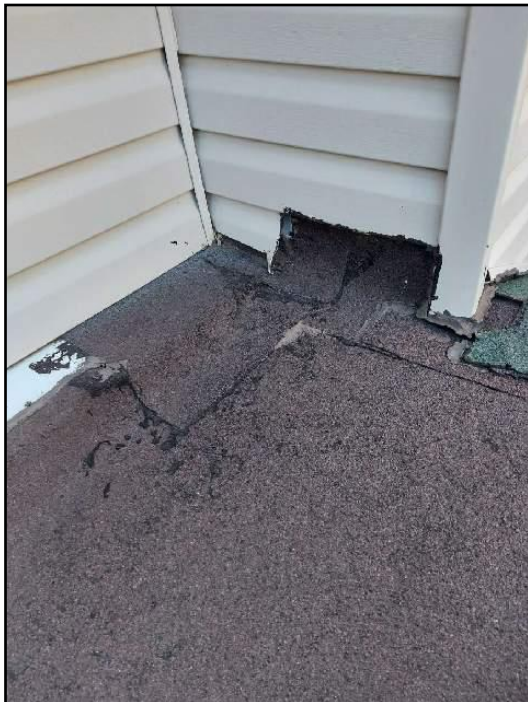
4. Missing flashing
