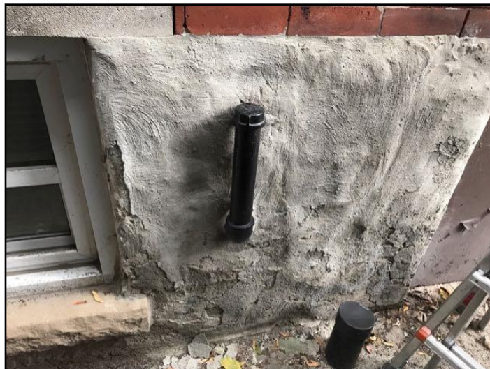
Fill pipe - abandoned
