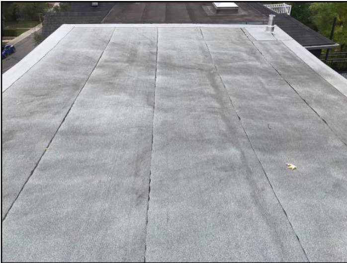
Modified bitumen membrane
