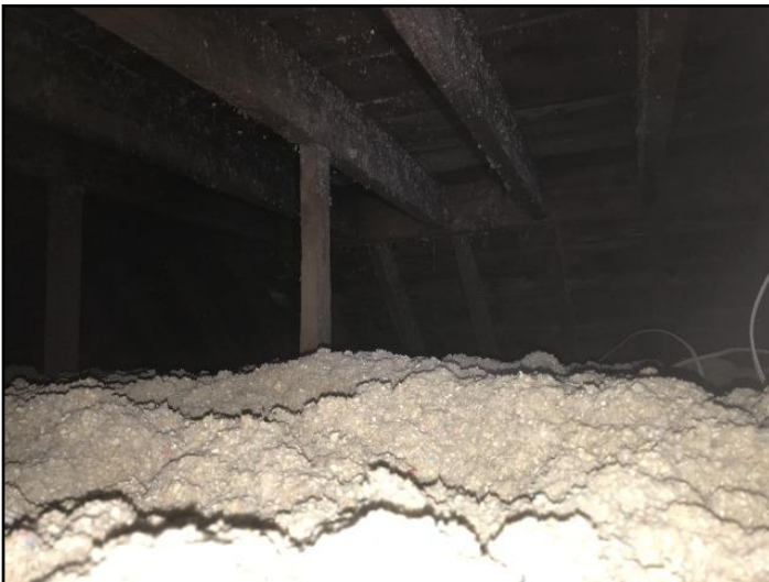
Inspected from access hatch
