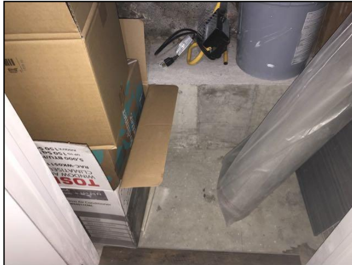
Interior drainage system - not visible...
