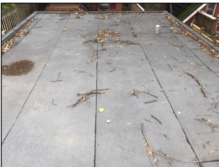
Modified bitumen membrane
