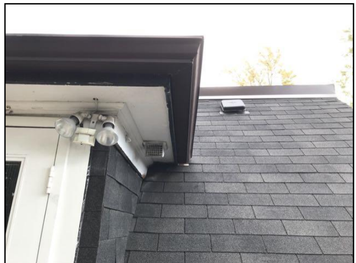
Discharges onto roof
