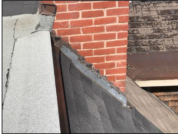
Flashing - patched
