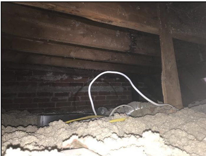
Inspected from access hatch
