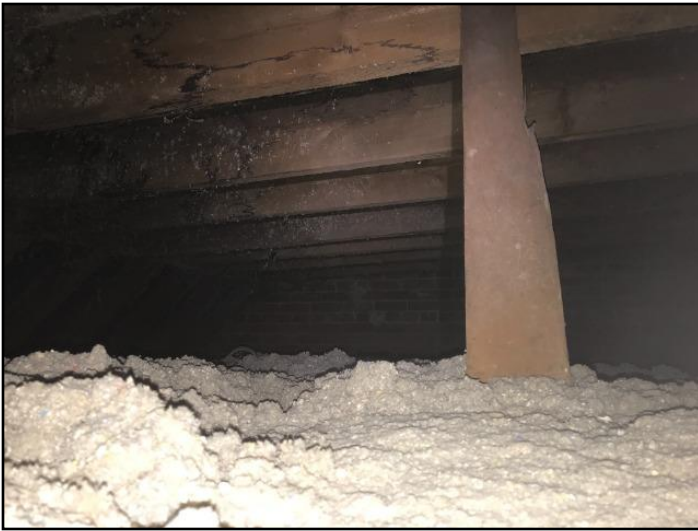
Inspected from access hatch
