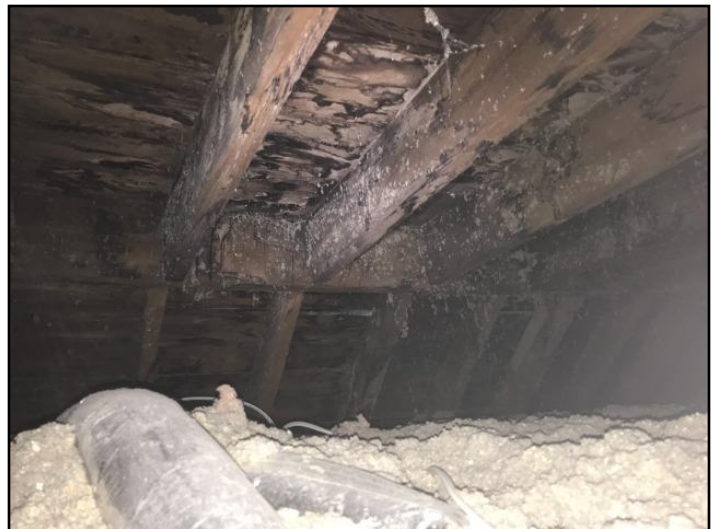
Inspected from access hatch
