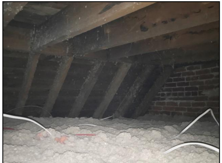
Inspected from access hatch
