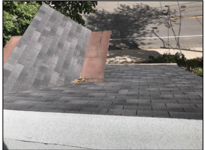
Asphalt shingles
