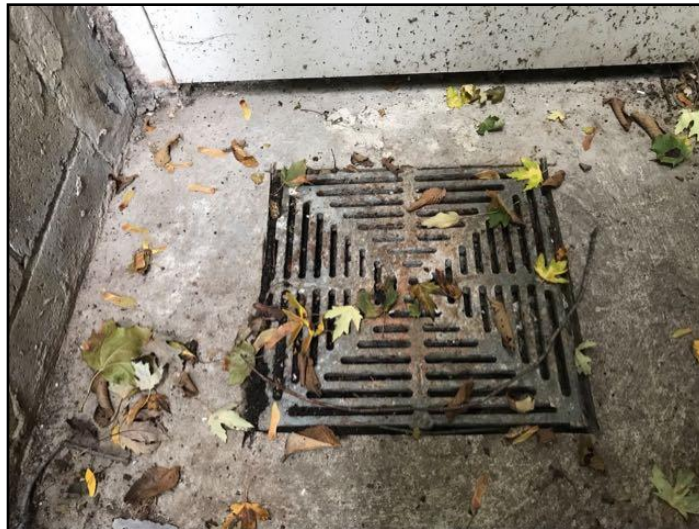
Floor drain - vulnerable area...
