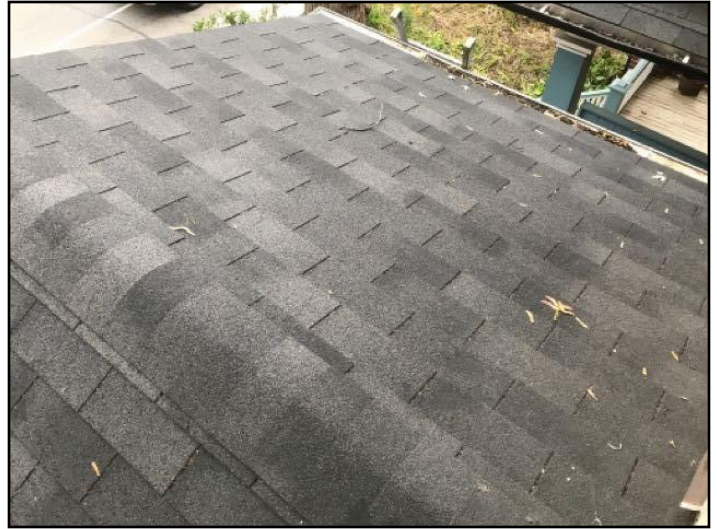
Asphalt shingles
