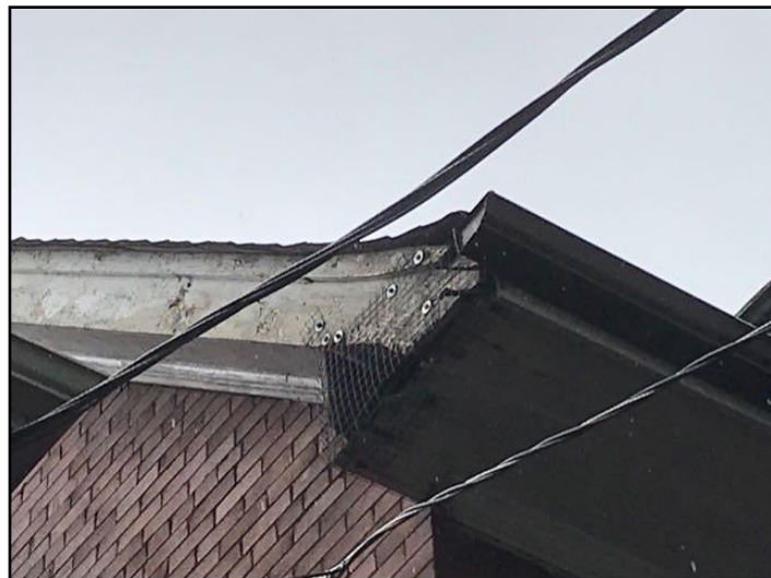
Water/vermin damage
