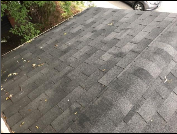
Asphalt shingles
