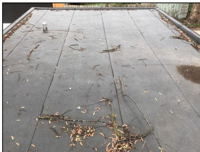
Modified bitumen membrane
