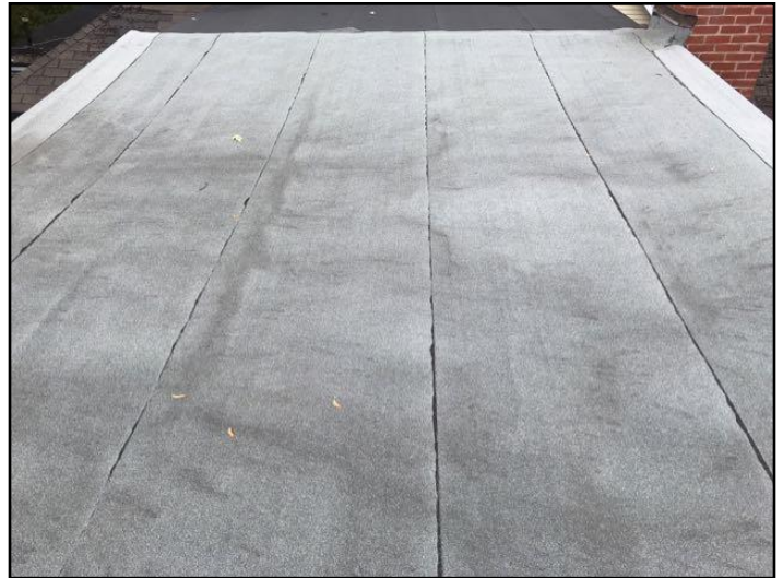
Modified bitumen membrane
