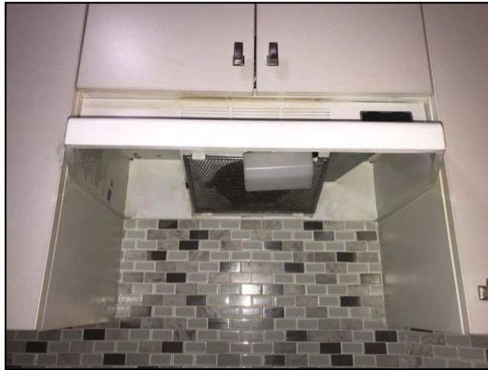
Baffle - missing
