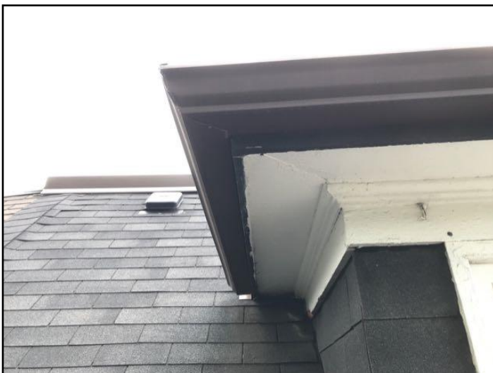
Discharges onto roof
