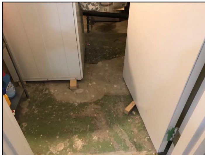
Floor drain - not visible
