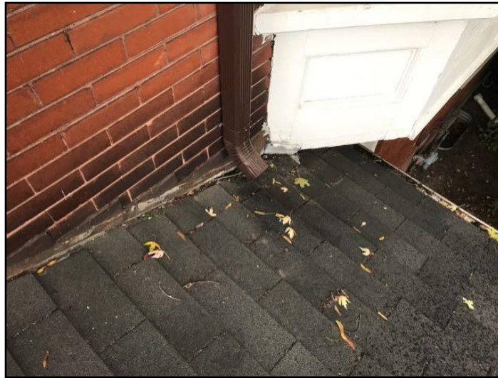
Discharges onto roof
