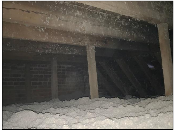
Inspected from access hatch
