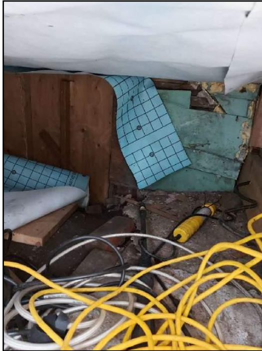
4. View of crawlspace
