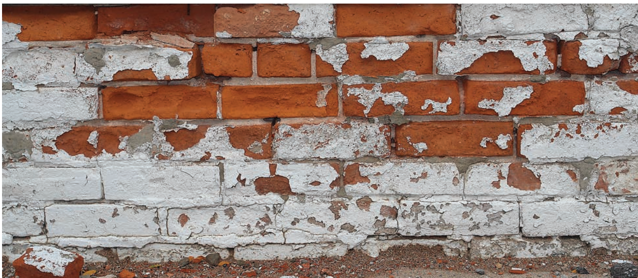
Brick Spalled by Retained Moisture
