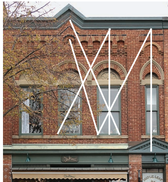
Control lines tie the diagonals and centre-lines of windows and piers to the decorative brickwork and set the height of the parapet
